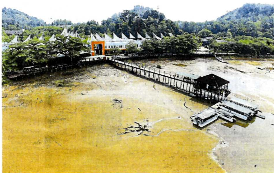
Dam-pened spirits: An aerial view of the dried up lake in Bukit Merah Laketown Resort in Kerian. — Drone photography by Se Vena Networks
