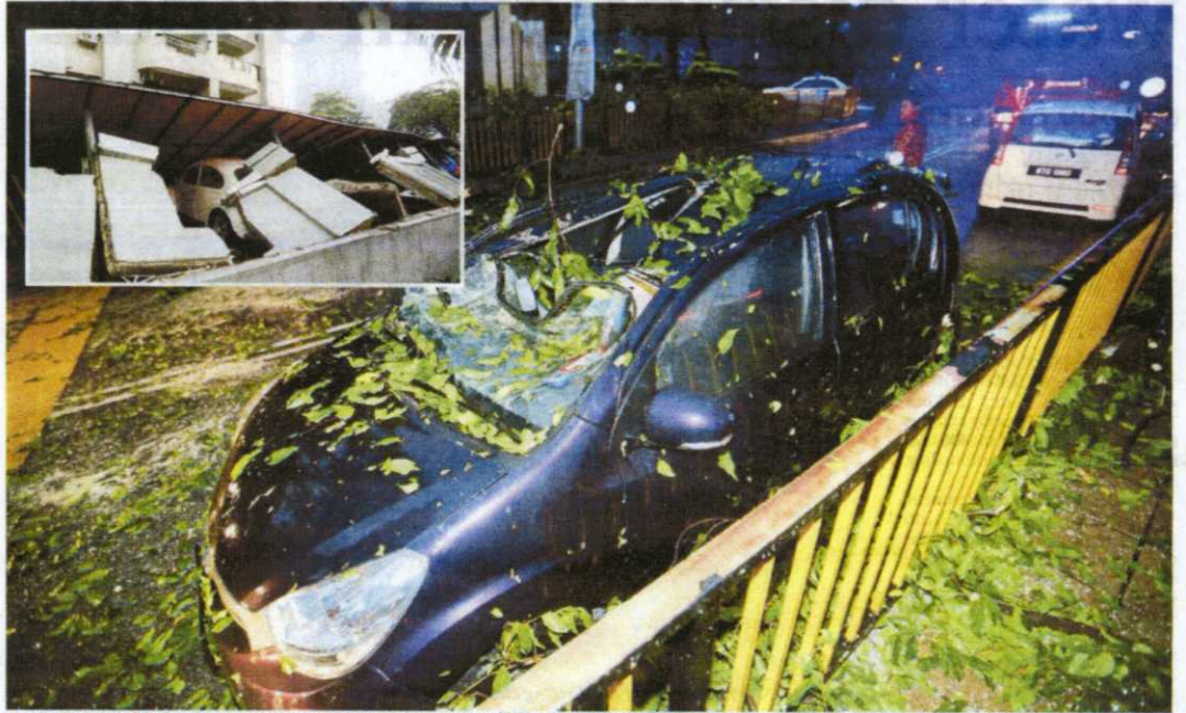
A car damaged by an uprooted tree near the Bank Negara komuter station in Kuala Lumpur yesterday. (Inset) One of the four cars that were damaged when the garage of an apartment collapsed in Bangsar, Kuala Lumpur, yesterday. Pix by Zulfadhli Zulkifli and Abdullah Yusof
