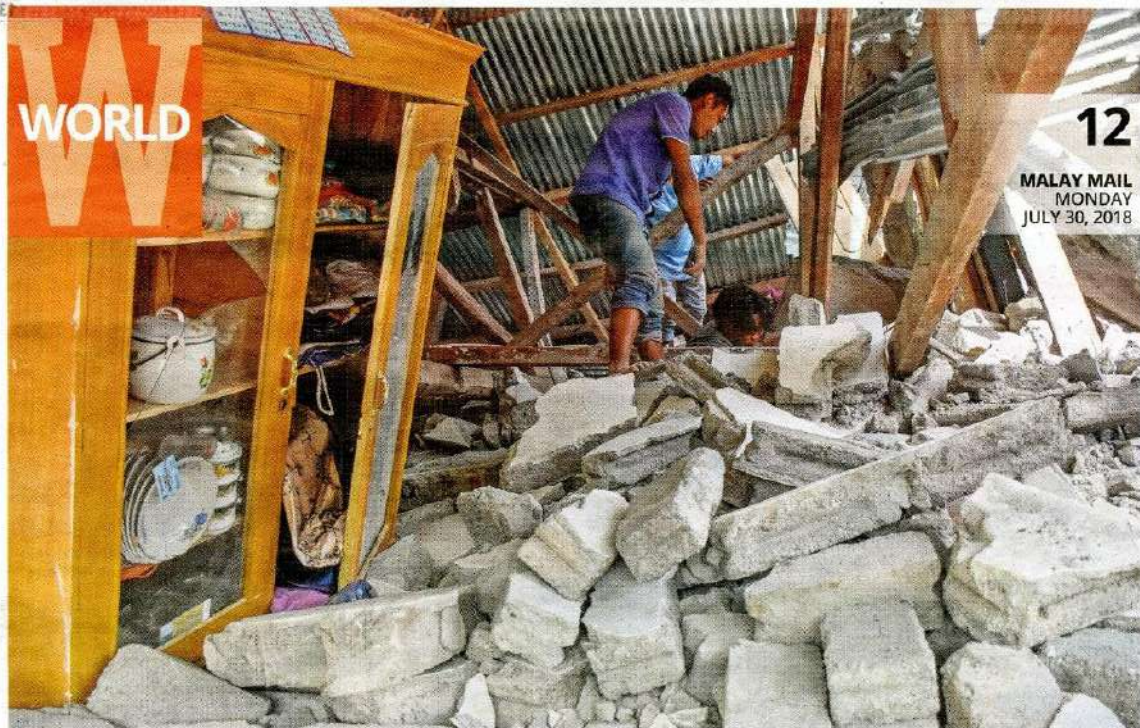
A villager walks through the ruins of a collapsed house at Sembalun Selong village in Lombok Timur. — Picture by Reuters
