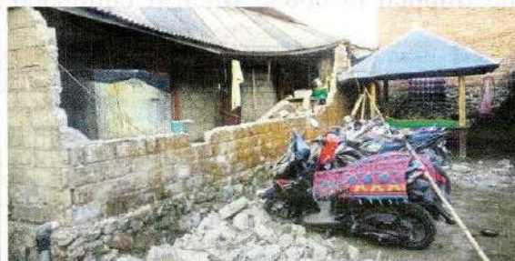
The damage caused by an earthquake in Lombok yesterday.
