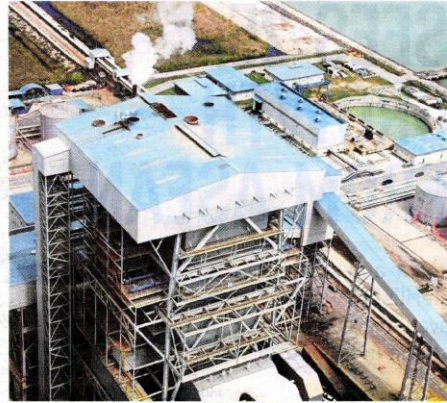
A Tenaga Nasional Manjung 5 plant. The national utility sources its coal overseas with over 60 per cent purchased from Indonesia.
