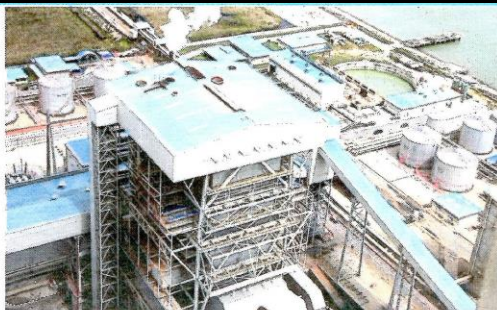
Malaysian power producers mostly depend on gas and coal for 90 per cent of their power generation needs.
